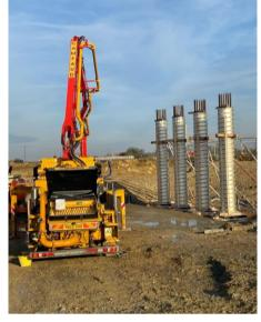
Shutters were then installed around the steel before concrete was poured and left to cure to form reinforced concrete columns. A blackjack waterproof coating has then been applied to create a waterproof barrier. Concrete sleeving is then installed which will allow the columns to flex when the bridge expands or contracts depending on temperatures.
