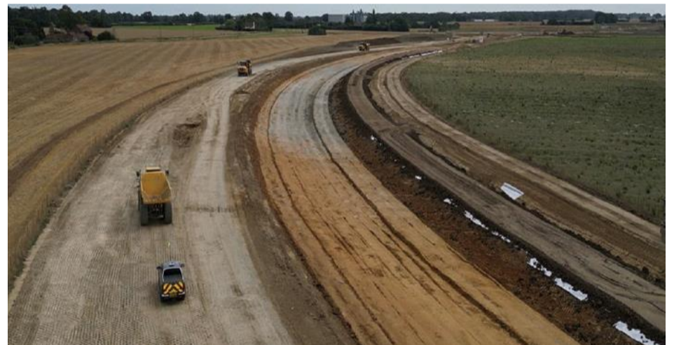
Cut ready for stabilisation trial & construction of environmental bund
