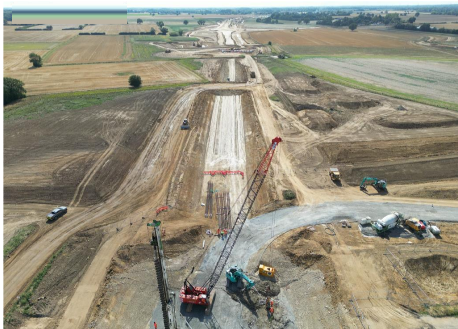
Hall Lane piling location, looking south
